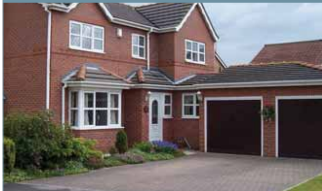
Front Doors & Office Doors; Garage Door/Roller Shutters
